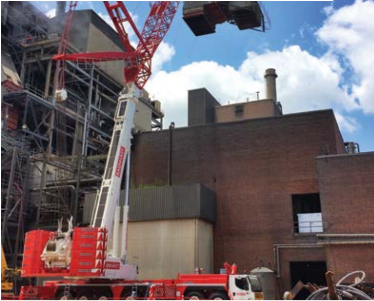
Barnhart removes precipitator ductwork with a 500T Liebherr at a papermill in Louisiana.
